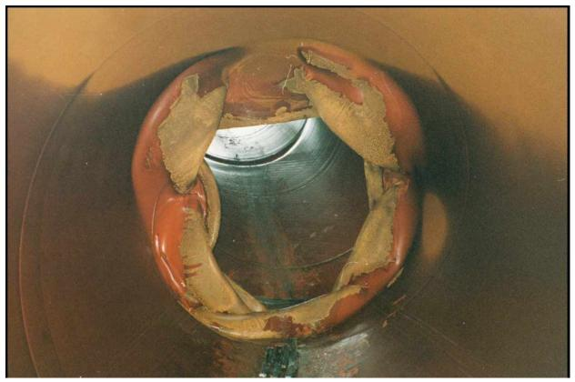
Figure 3. Major Wrinkle. Remaining Flow Diameter is 1400 mm
