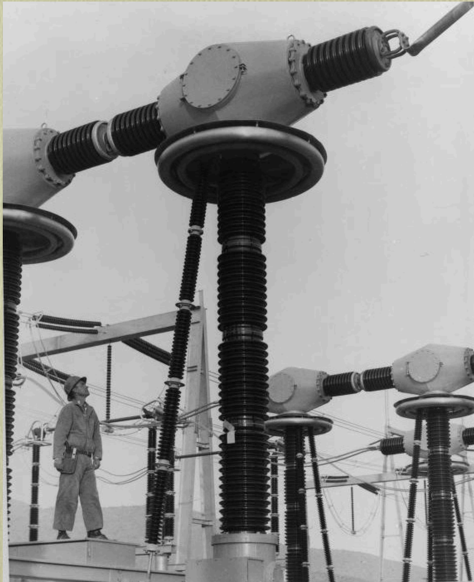
Westinghouse 500 kV CBs being installed at Vincent Substation (c. 1968).
