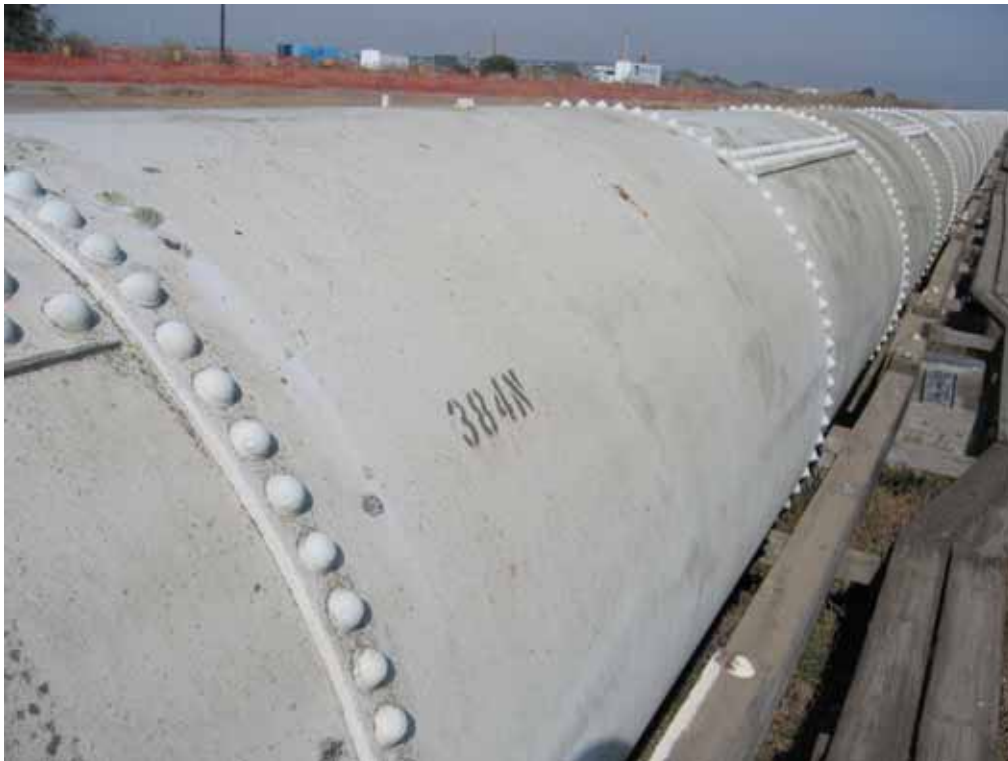
Figure 8-2. 60" Diameter Riveted Steel Pipe (Built 1925)
