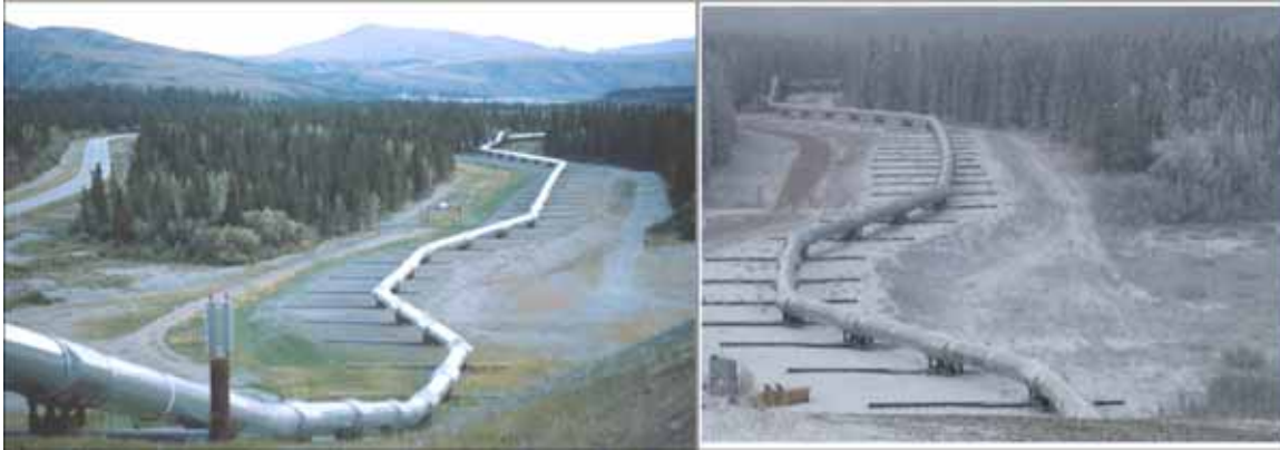
Figure 8-14. Alyeska Pipeline At Denali Fault (Left = before, Right = after)
